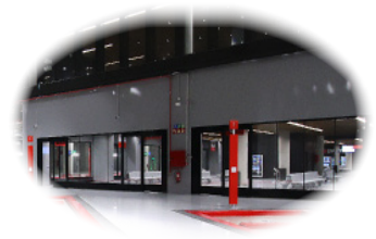
Interchange bus station (Termibus - Bilbao)
