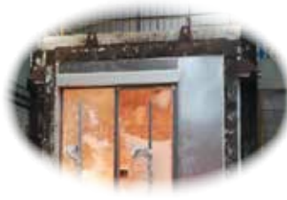
Fire proof glazed sliding door EW60 rating
